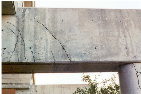
Figure 4: Diagonal cracks in the beam
