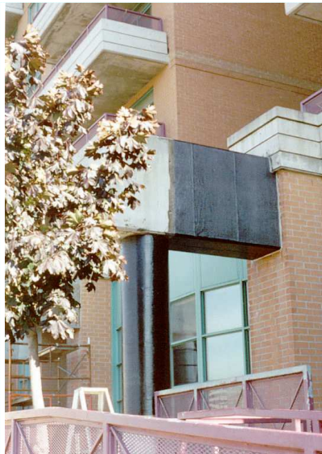
Figure 7: Structure retrofitted with CFRP
