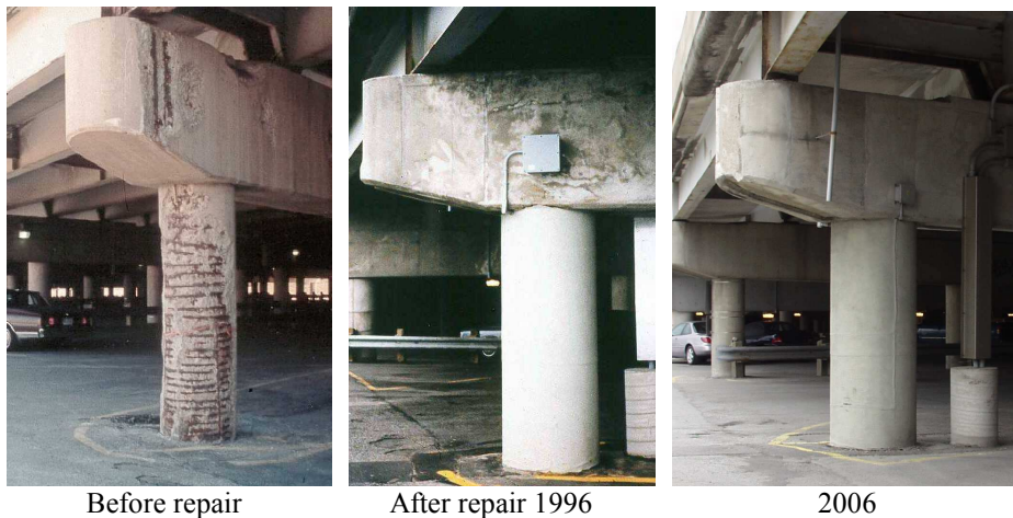
Figure 5. Columns before and after repair
