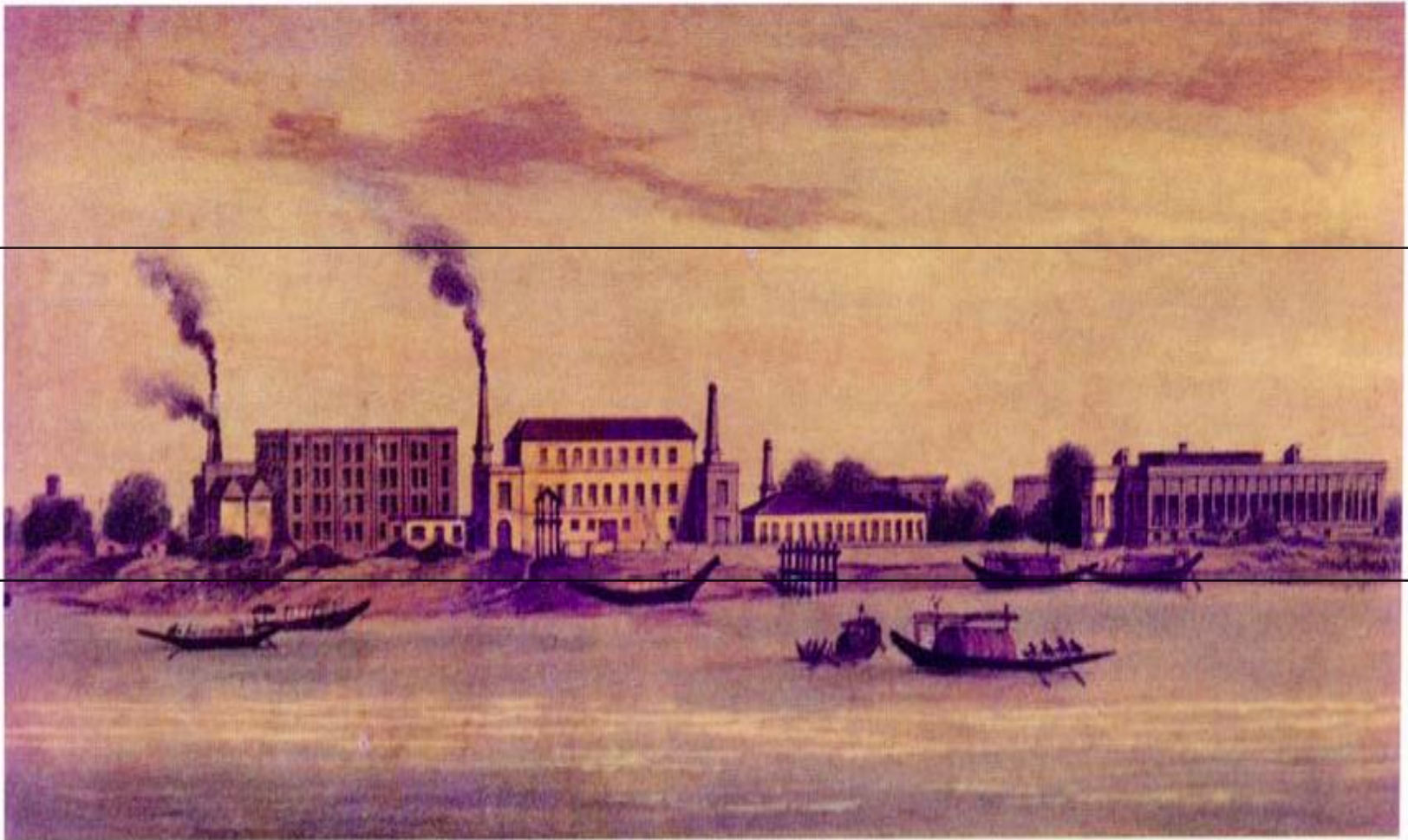
The Dhaka Sugar Company works (popularly known as the mill barracks) and the manager's residence
